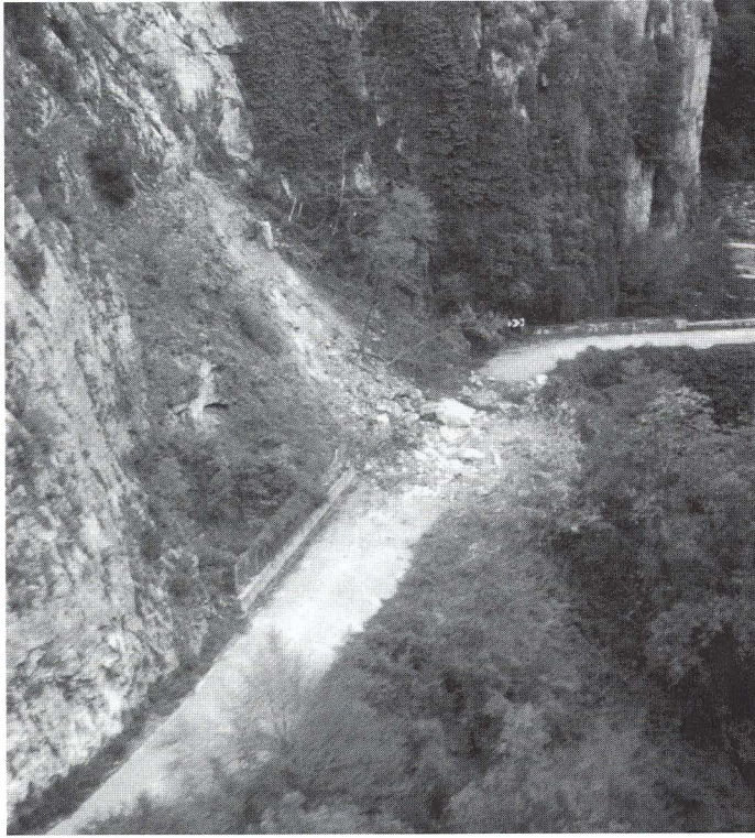
Fig. 6 - Corno Valley, near Triponzo. Examples of an earthquake induced rockslide along a dismissed road. The 14 October 1997 earthquake triggered the landslide.
