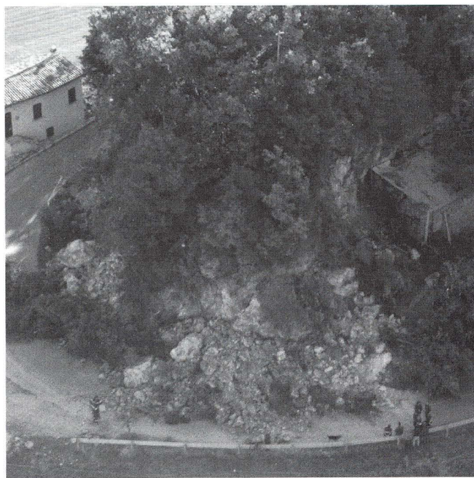
Fig. 7 - Stravignano. Examples of an earthquake-induced rock topple along a road. The travertine cap failed during the night of 16-17 October 1997, and was the result of the cumulative effect of ground shaking produced by several aftershocks.
