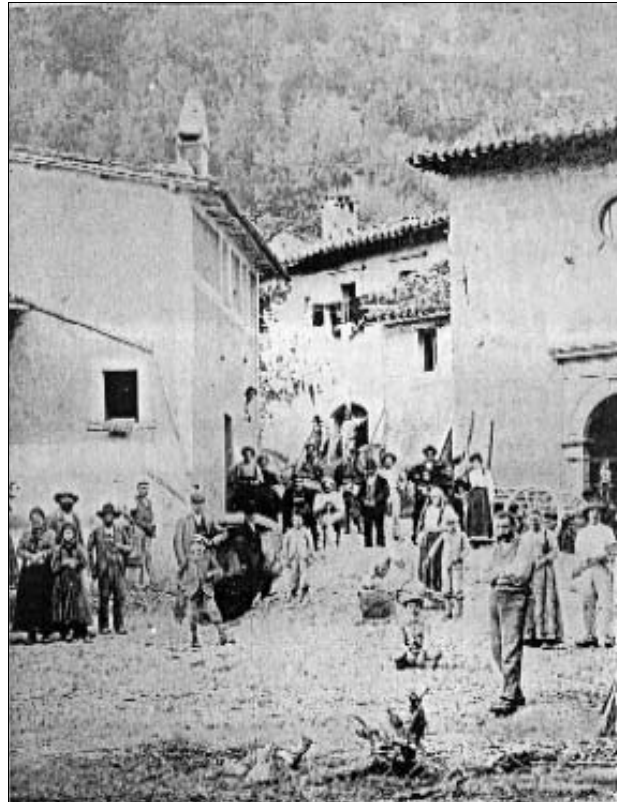
Figure 1. The village of Castel Sant'Angelo sul Nera inundated by a debris flow on 27 July 1906.
